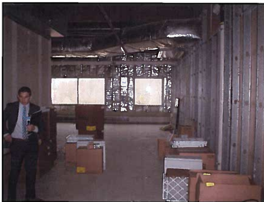
View of the vacant "shell" space on the third floor.
