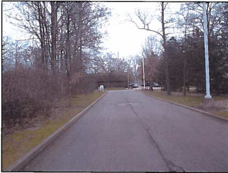
View of the access drive to First Street looking north.
