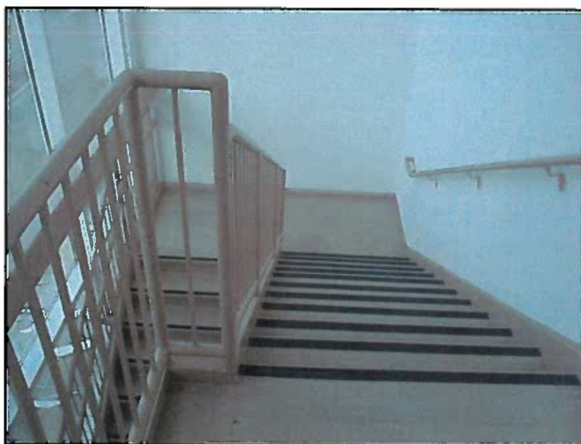
View of a typical stairwell.
