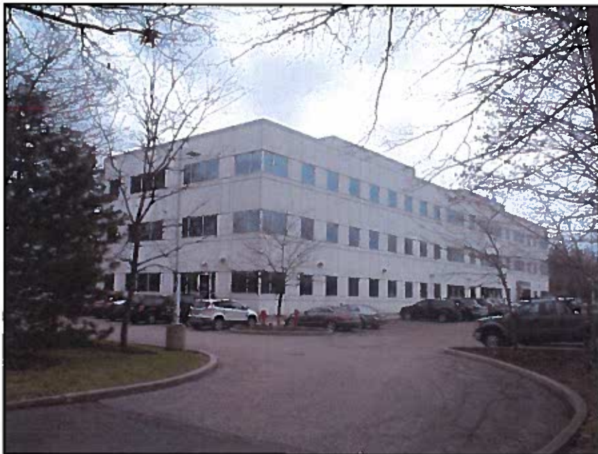
View looking southeast from a point near the subject's access drive from First Street.
