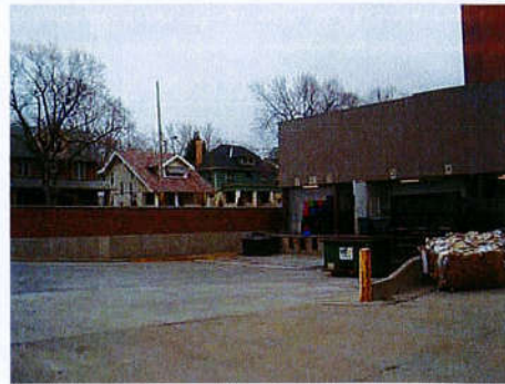
Figure 7: View of loading area
