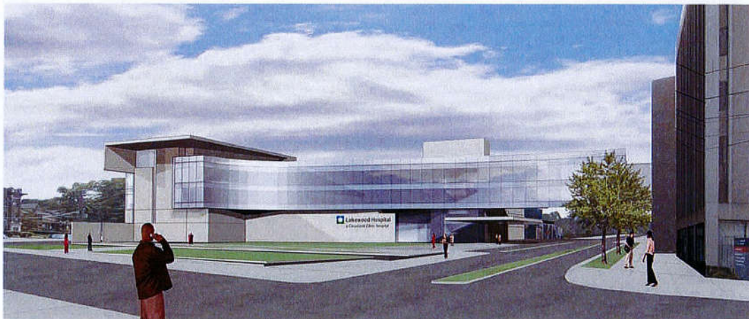
Figure 12: View of new addition from Detroit Avenue showing new entry and landscaping.
